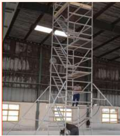
14M working height Scaffolding delivered to IT company
